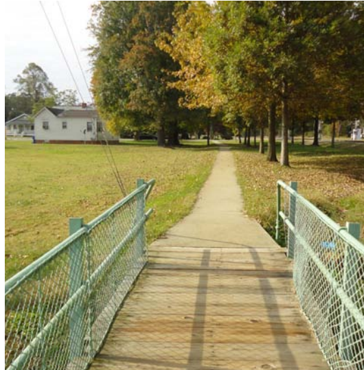
Pedestrian bridge connection over Whitsett Street.
