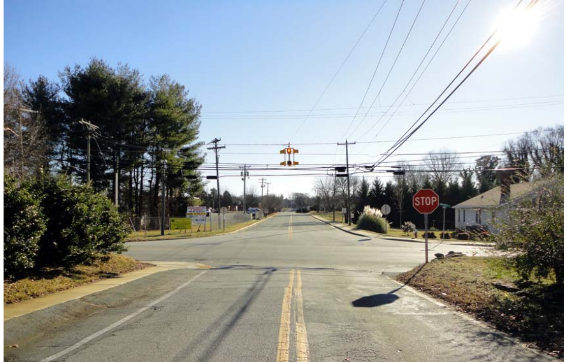
Minneola Street and Whitsett Street existing conditions
