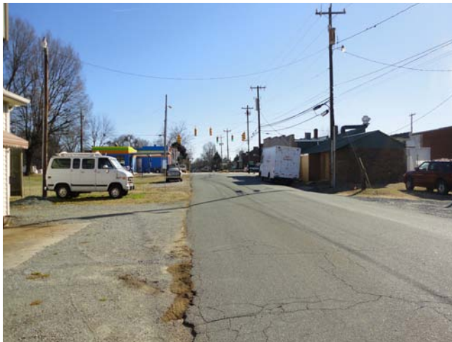
A gap in the sidewalk network along Burlington Avenue as it approaches Lewis Street forces pedestrians to walk through a parking lot and grass area.
